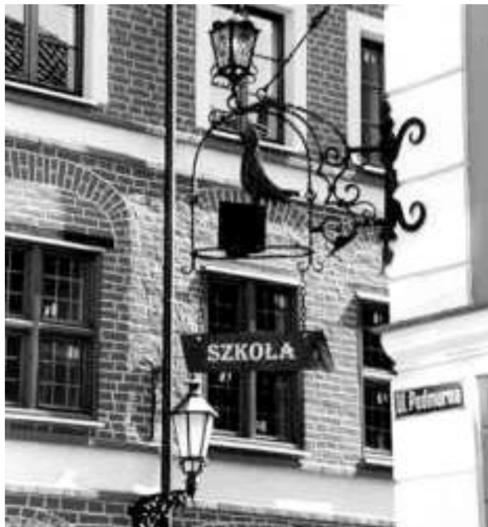
stara szkoła. old school in the old part of Toruń
